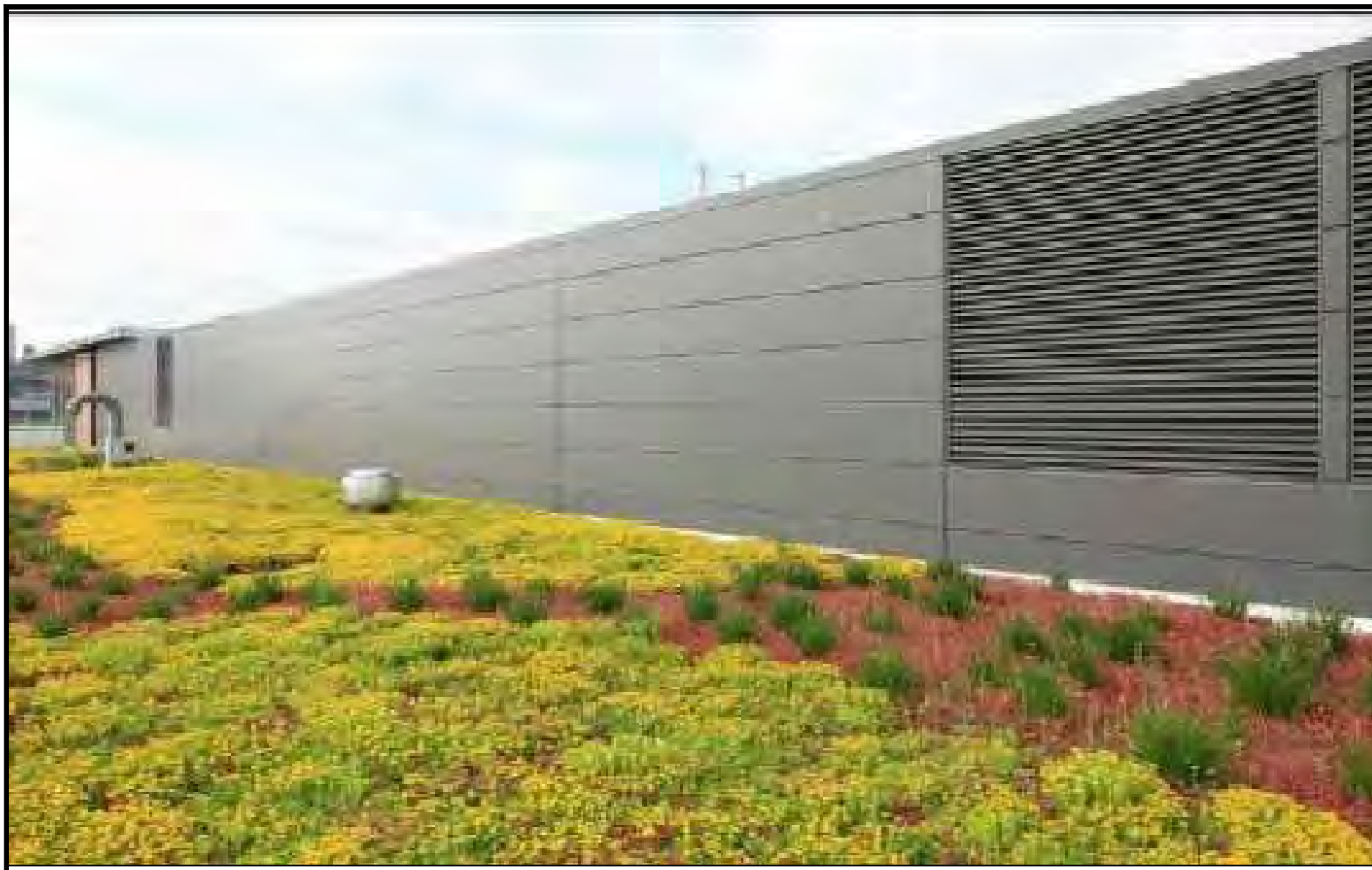
A. GREEN ROOF
